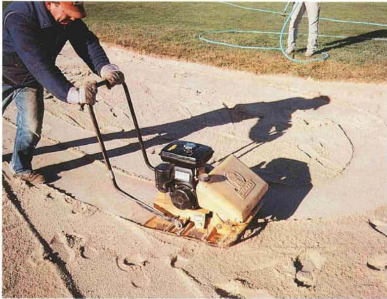
A cement finisher has proven to be an ideal tool for firming new sand in recently renovated bunkers at the Bridgehampton Club.
