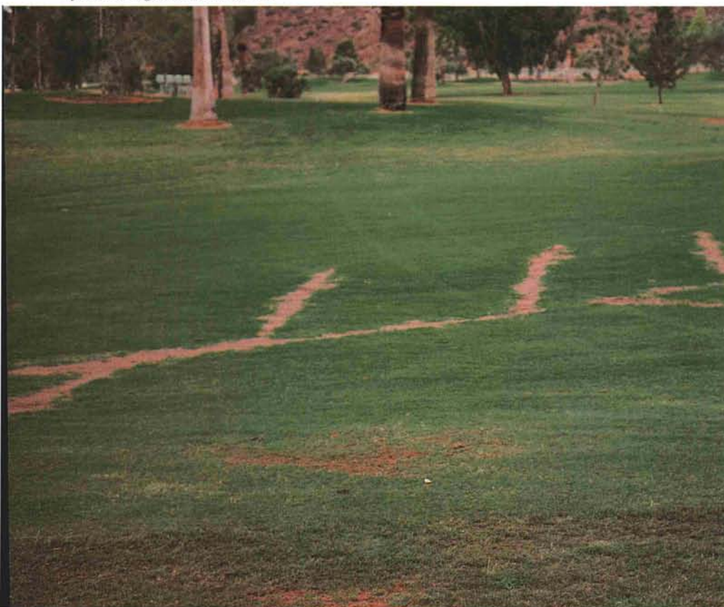
Basic subsurface drainage tile installation is still the most important means of removing excess moisture.
