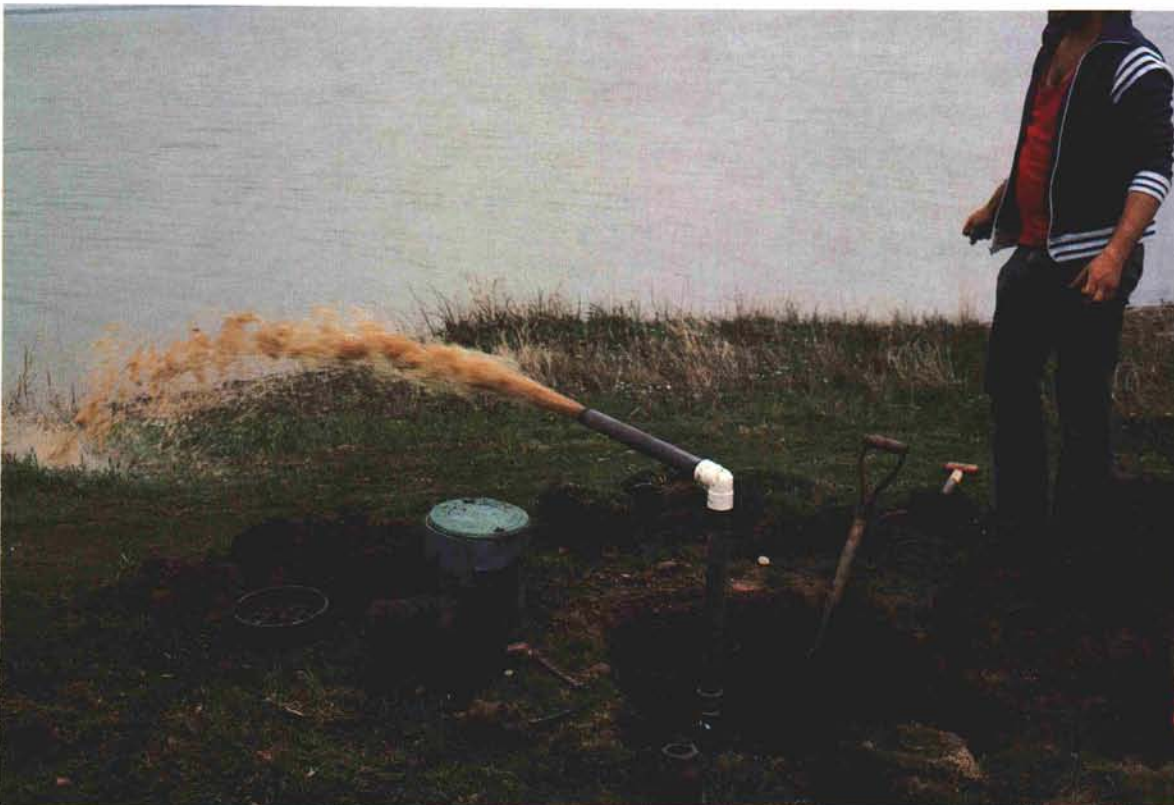
Water quality must also be closely evaluated. The sediment in this water could ruin even the best green in a few short seasons.
