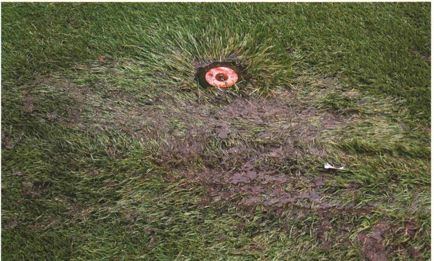
With a zone or block system, the low sprinkler heads in each zone can weep, creating obvious problems.
