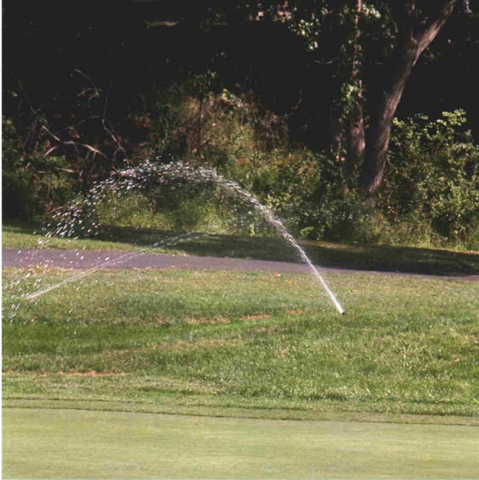
Too many sprinklers on one line spell insufficient pressure and poor coverage.
