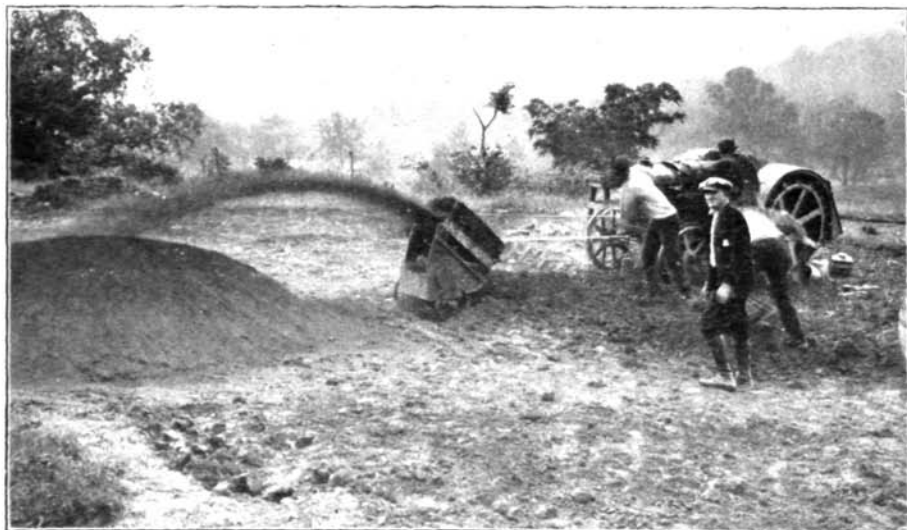
A compost and soil sifting machine which was tried out during the season of 1924. It is claimed that this machine in one case screened more top soil at a labor cost of $15.50 than was screened through a rotary screen by 5 men over a period of 3 weeks, at a labor cost of $455.
