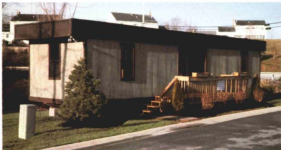
Prefabricated trailers provide a viable option as interim office space.
