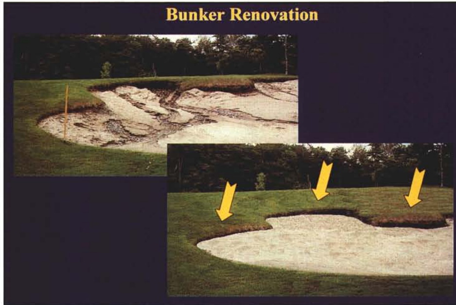
Addressing the fear of the unknown with computer imaging can be a very useful tool for presenting project proposals. To show golfers that lowering the sod line on eroding bunker faces will not significantly alter their appearance, digital images can be downloaded onto a computer and easily manipulated.
