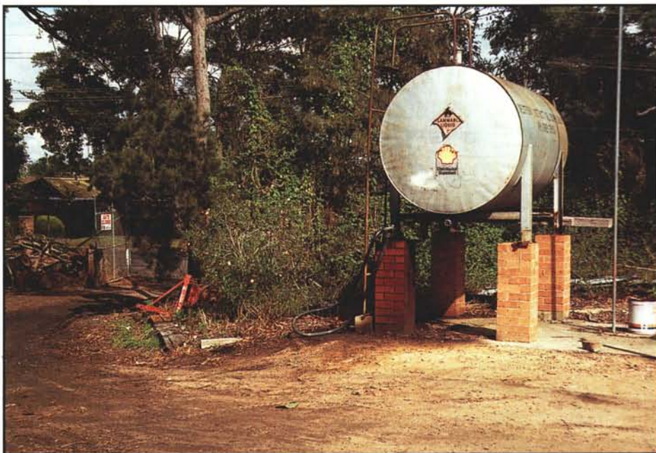
Fuel storage is a major environmental issue for most golf courses. Containment for the storage containers is becoming a basic minimum to reduce the potential for environmental damage.
