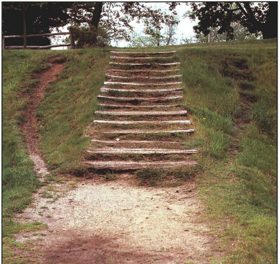
Obviously, this well-worn path is a sure sign that these steps aren't in good enough condition for golfers to use.
