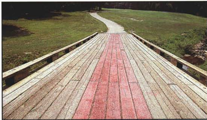
A combination of fast-drying epoxy paint and sand-blasting material can be used to create and preserve a textured surface. When the combination dries, the surface is wear tolerant, aesthetically acceptable, and coarse textured.
