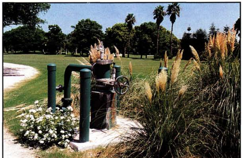
A 1,500-foot-deep artesian well supplies brackish water to the reverse osmosis plant at the Jupiter Island Club (Jupiter, Florida).
