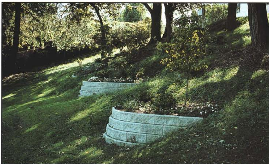
The crew gained valuable hands-on experience when they cleaned up the hillside adjacent to the sixth green and also installed brick planters, which improved the aesthetic quality of the hole (McCall Field Golf Club, Upper Darby, Pennsylvania).
