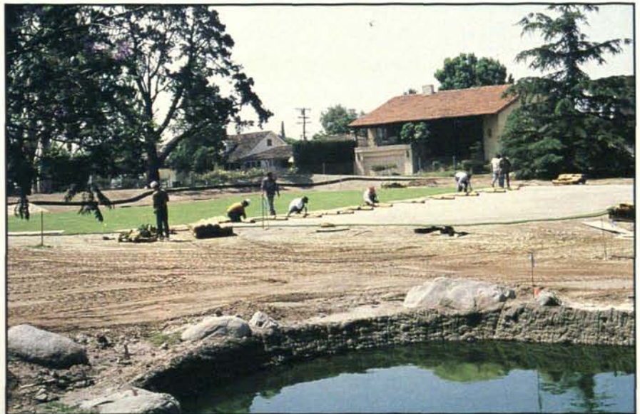
The decision was made to sod the tees, greens, and fairways. This was a controversial decision for the city, but sodding allowed the golf course to open five months early. The additional revenue that was generated by opening early easily offset the cost of the sod.
